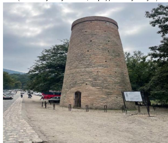
Fig. 4: Water pressure relief tower, By Authors
